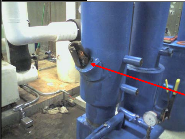
Defective Water Valve
